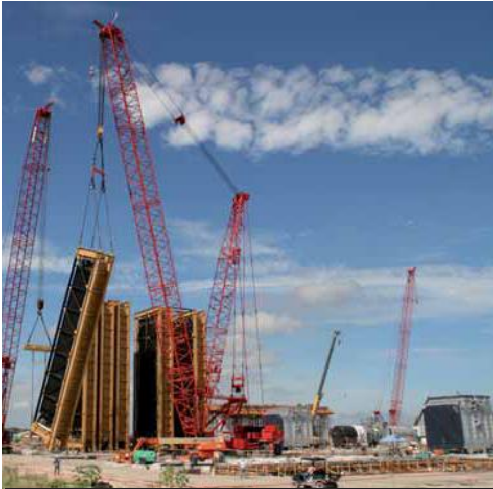
CRC used two Manitowoc Model 2250 crawler cranes to lift and place 40 boiler units
